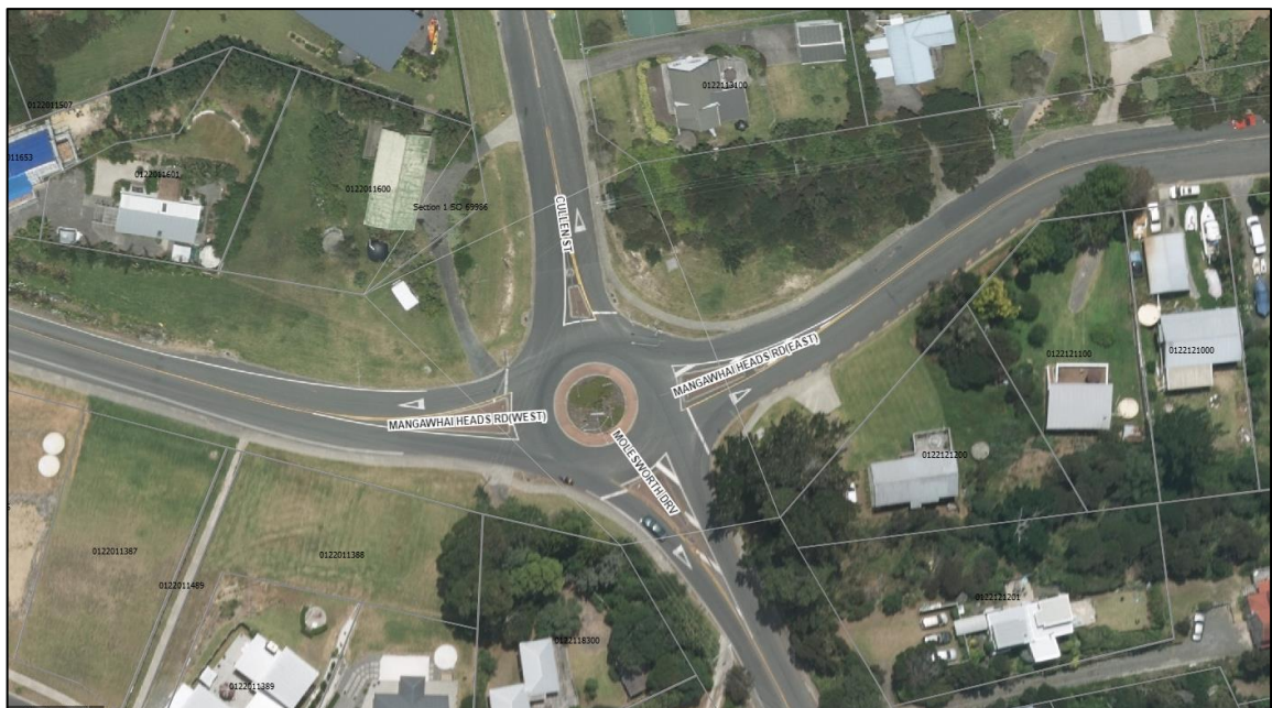
Figure 24: Mangawhai Heads Road – Cullen Street – Molesworth Drive Roundabout Image Source: Kaipara District Council's GIS maps
